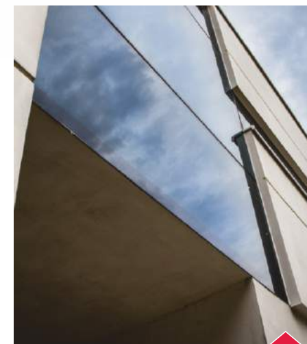
One of the options is a facade without visible profiles (SL solution)
