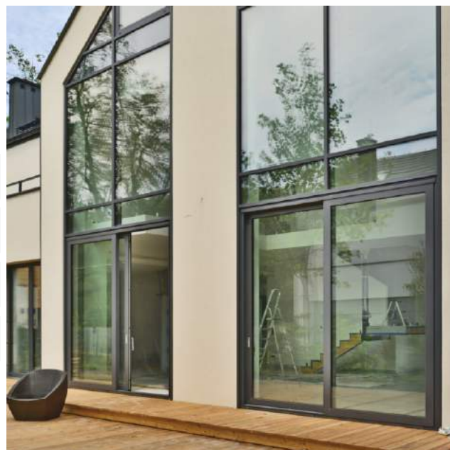
One of the options is a facade without visible profiles (SL solution)
